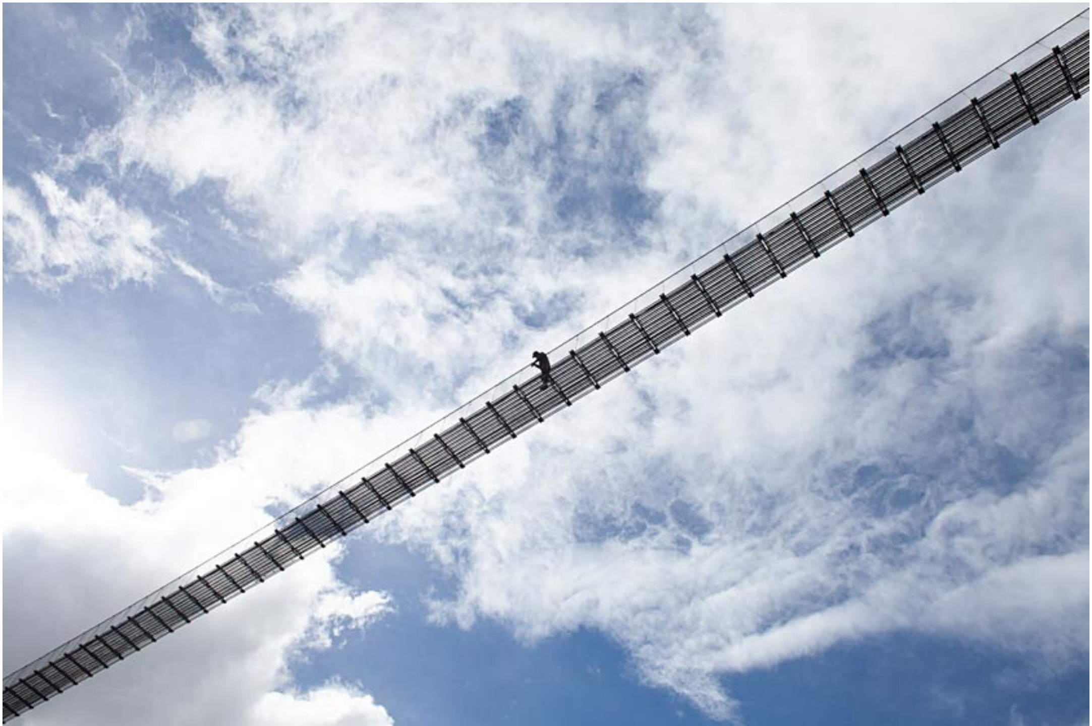
MAN REPAIRS A BRIDGE IN EVEREST
